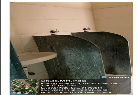
Toilet for Boys 1
